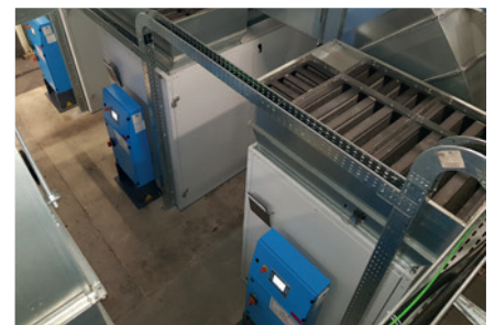
BAUER high pressure compressors deliver the necessary pressure to the presses.
