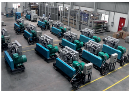
13 high-powered BAUER IK 28 compressors provide a reliable supply of compressed air
