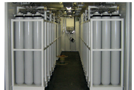
Vast racks of storage cylinders ensure permanent availability of breathing air.
